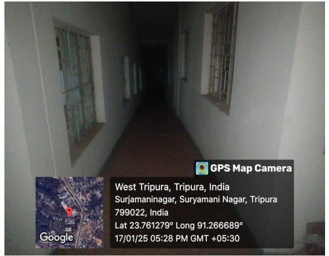
Disabled friendly Ramps in the department of Library Sciences, Tripura University
