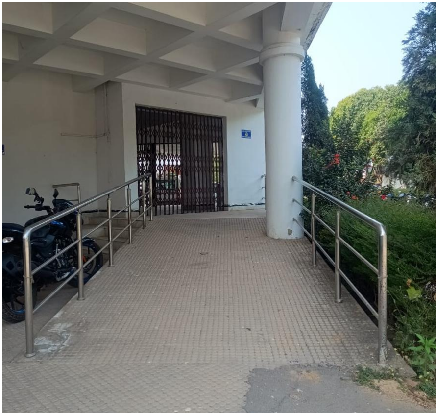
Disabled friendly Ramps, at the Examination building, Tripura University
