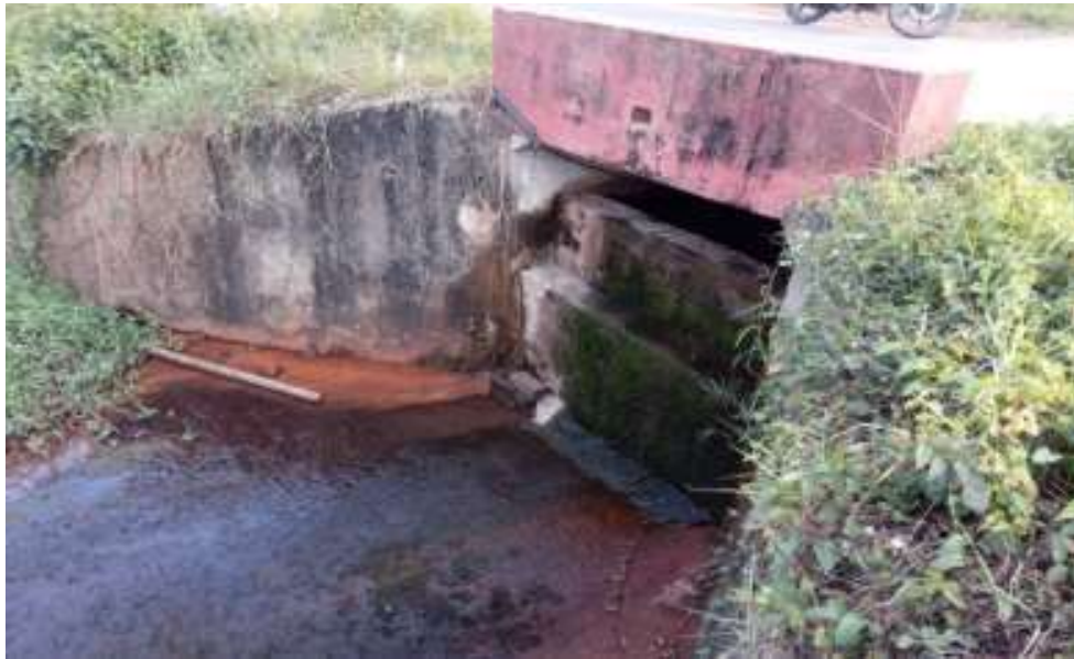
Photographs of sluice gate and semi permanent structure for conservation of water in Tripura University.
